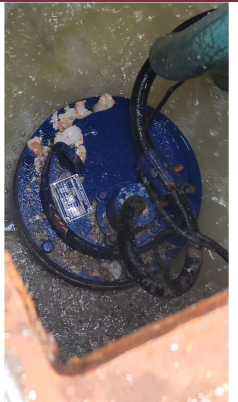
GPM-Eliminator pump in egg processing waste sump
