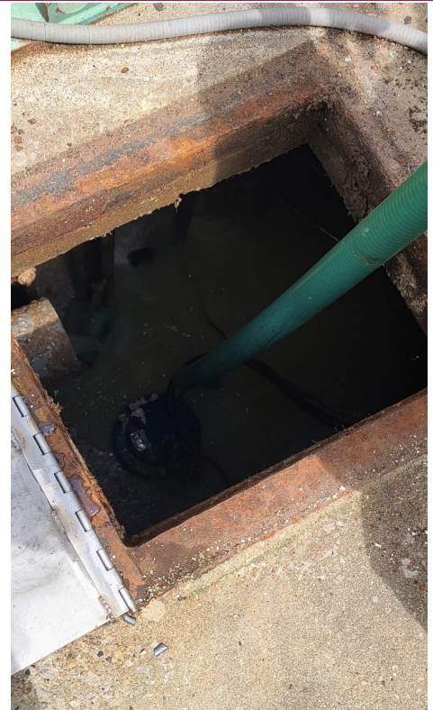
GPM-Eliminator pump in egg processing waste sump
